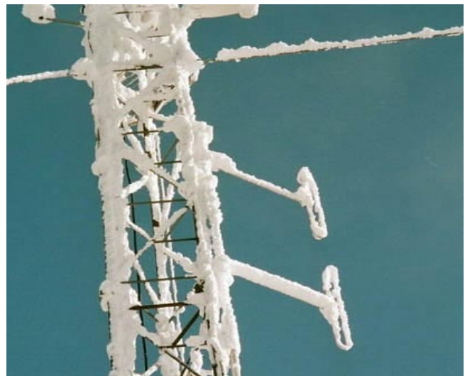
The WB1GQR repeater antenna coated with a thick layer of rime ice, making for treacherous winter maintenance
