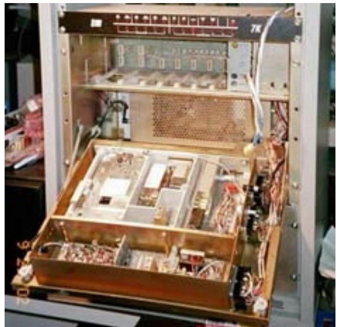
Opened up view of new repeater
